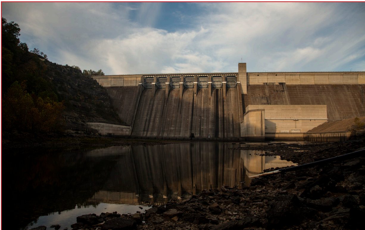
The Beaver Dam power plant operates two main 56 megawatt turbines and one house unit. The revenue from power generation is returned to the U.S Treasury to pay for the purchase price of the dam and the generating equipment Operations and Maintenance. (USACE Little Rock District photo)
